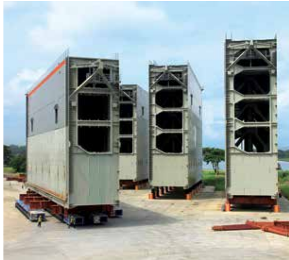
The new rolling gates range in height from 22.28 m to 33.04 m, depending on location.
